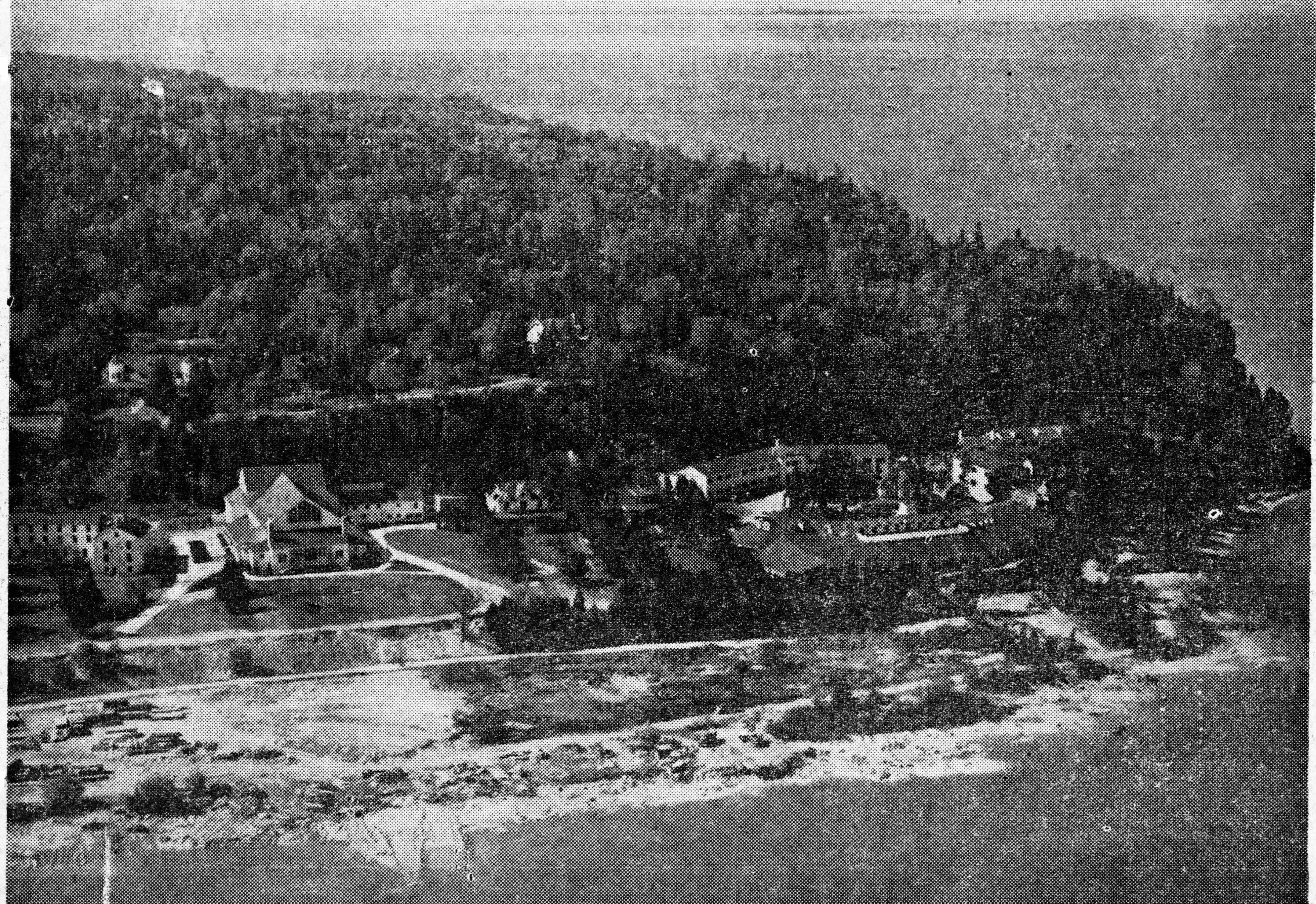
SITE OF THE ASSEMBLY OF NATIONS. The new buildings at Mackinac Island, Michigan, where delegates from every continent will meet beginning May 30. The Conference will continue through the summer. Historic Mackinac Island, lying at the heart of the Great Lakes, still retains the charm of horse-drawn carriages as the only means of transportation used.
