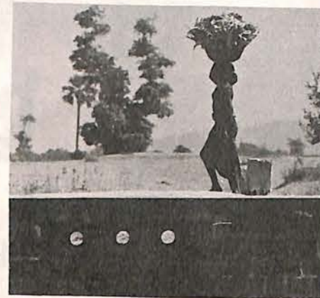
Lakhs of culverts allow roads to pass over small streams. If the tunnels are sealed after the rains and small holes left open at the top for surplus water to flow through, millions of gallons can be stored. Crops and wells come to life.
