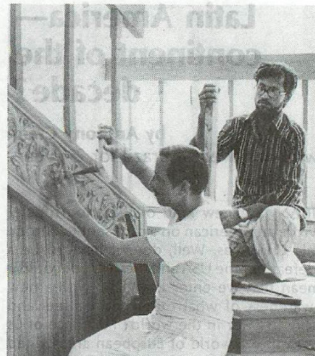
Carpenters at work on the staircase.
