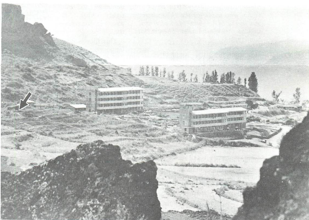
Asia Plateau, MRA world conference centre. Arrow points where theatre will be constructed photo Hartnell
