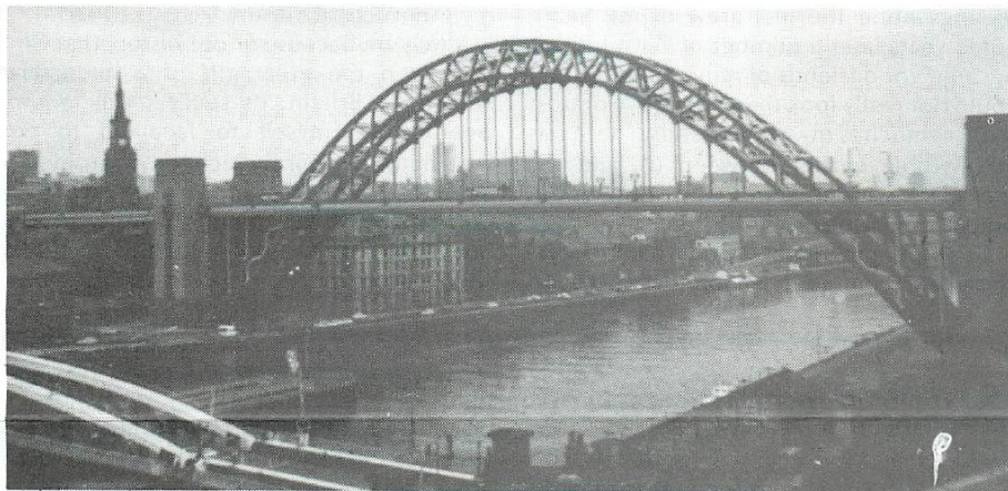
Bridge over the Tyne, Newcastle upon Tyne
