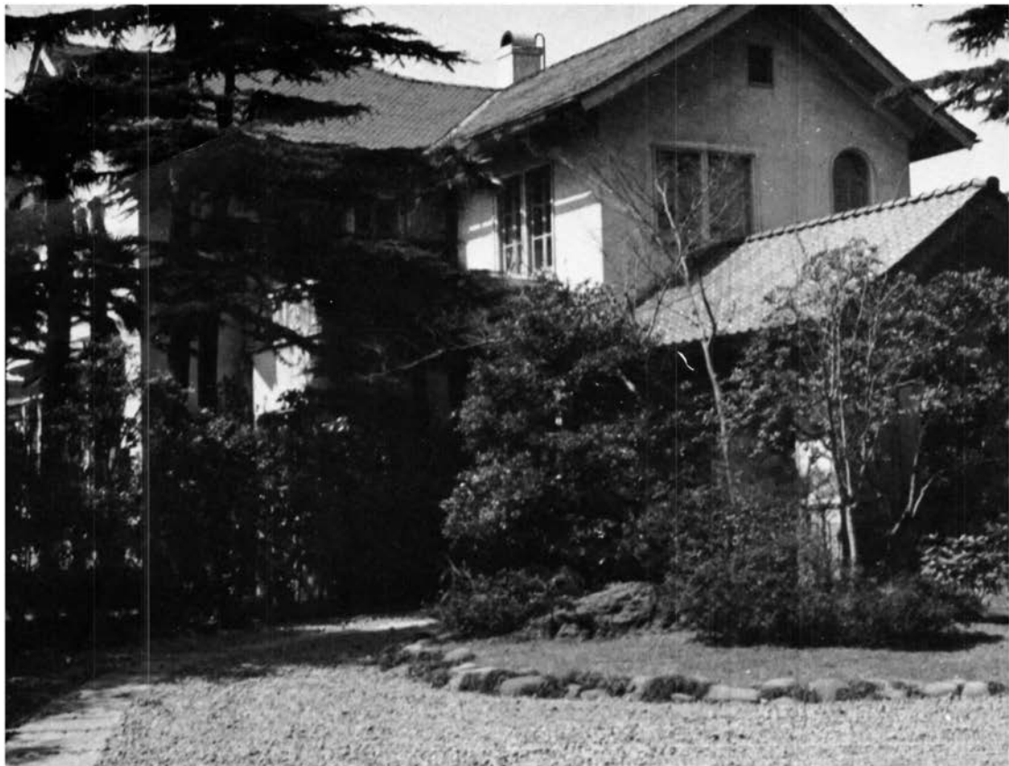
MRA House in Tokyo
