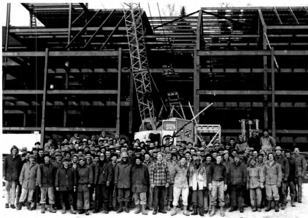
Construction crew, film studio
