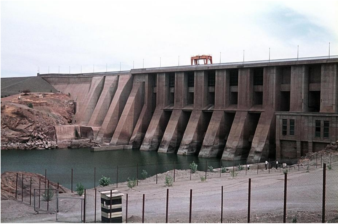
Dam at Khashm El Girba
