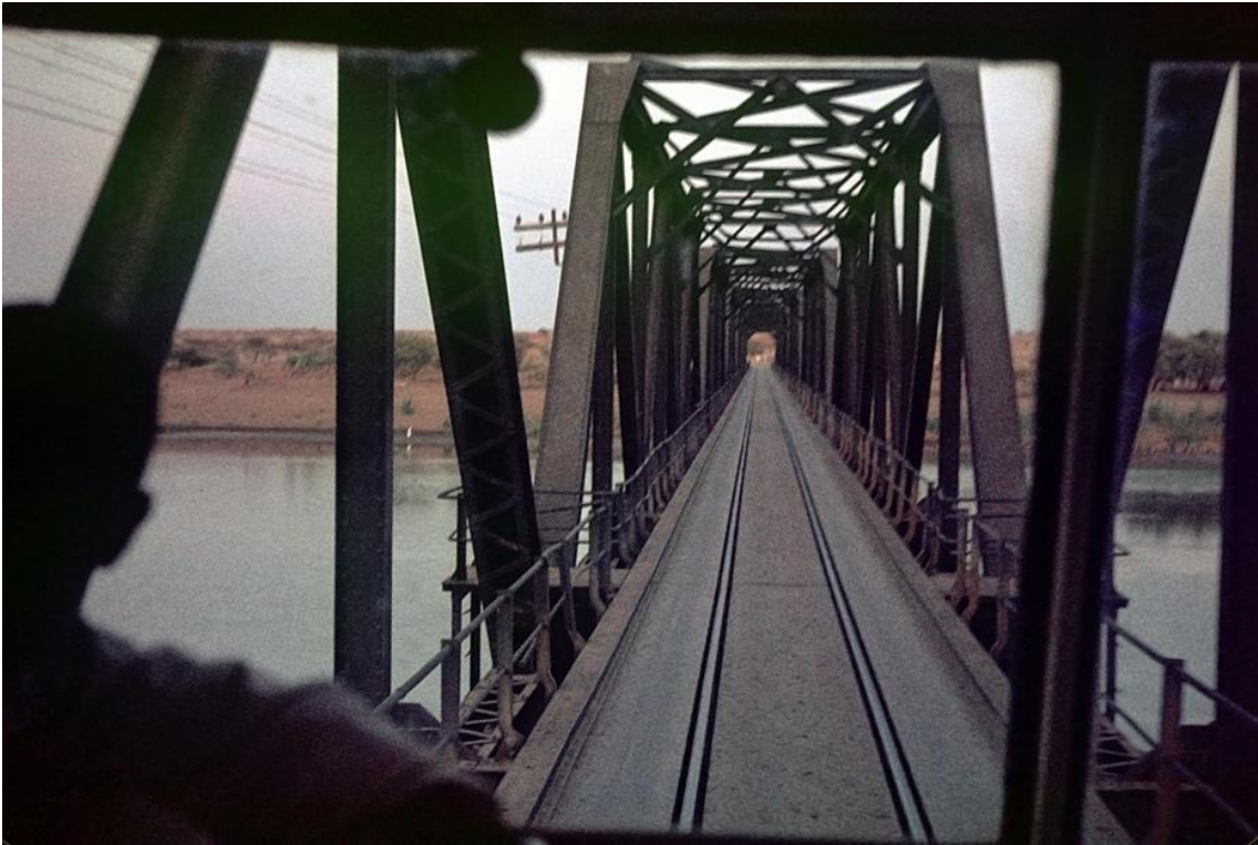
Bridge over River Atbara
