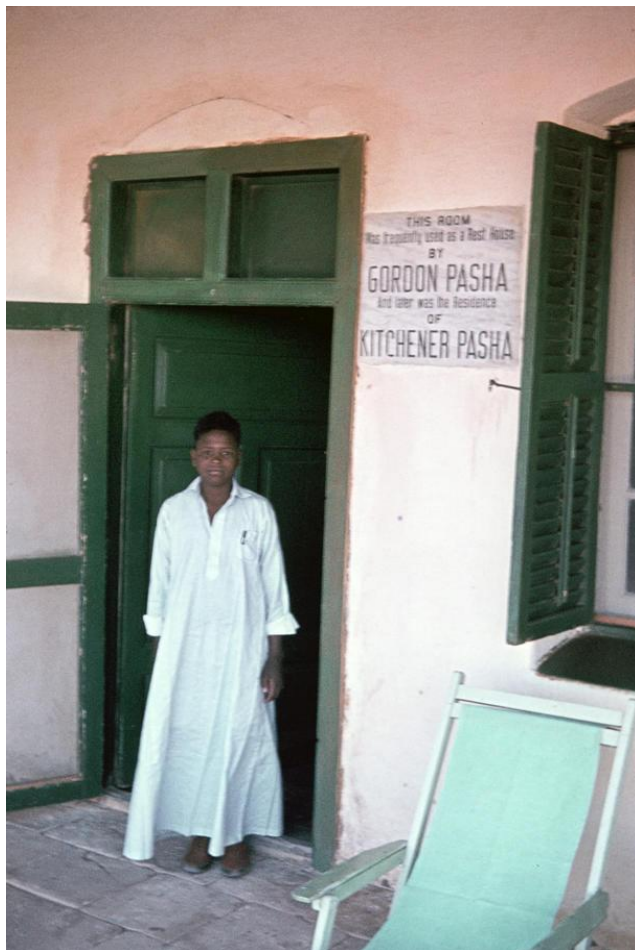
Resthouse at Halfa
