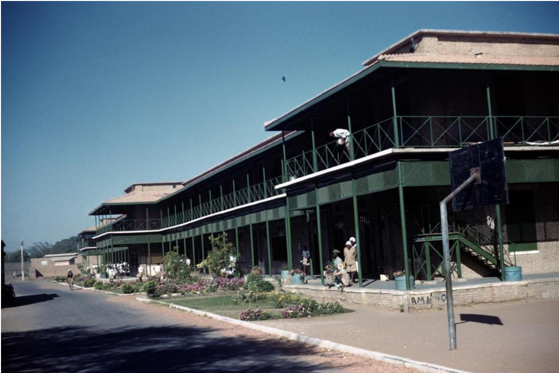
Khartoum Boys Secondary main building, former South Barracks
