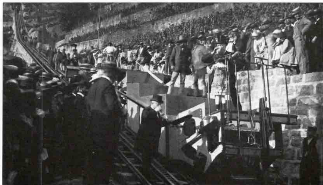
Safety test of the Territet-Glion funicular railway
