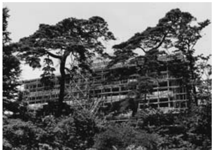
View from the southeast side
