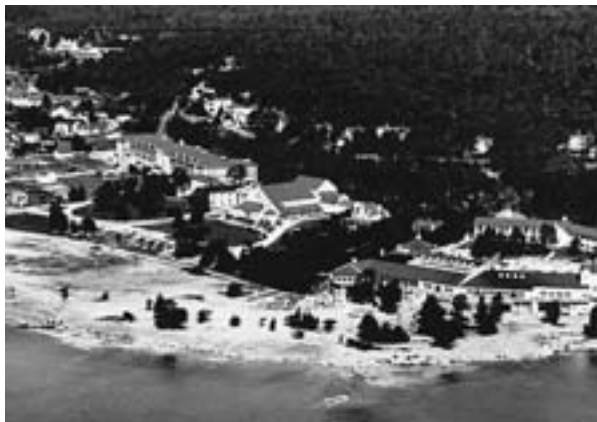
Bird's-eye view of the MRA headquarters on Mackinac Island
