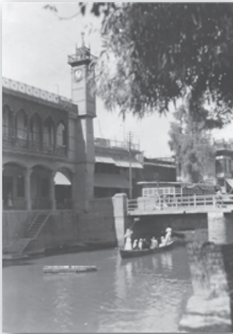
Ashar Creek, near the mission compound
