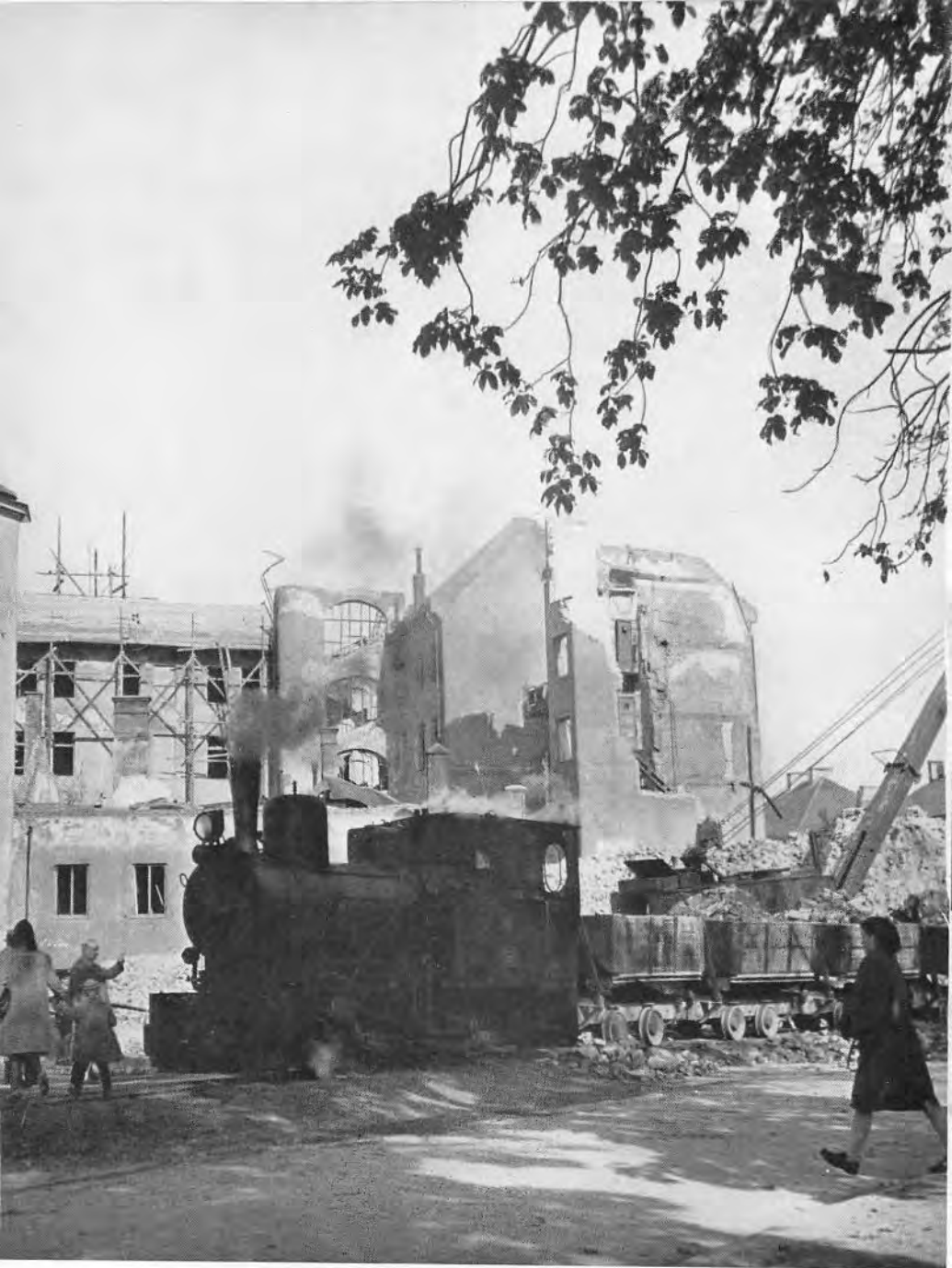
THE RUBBLE IS BEING CLEARED AWAY
