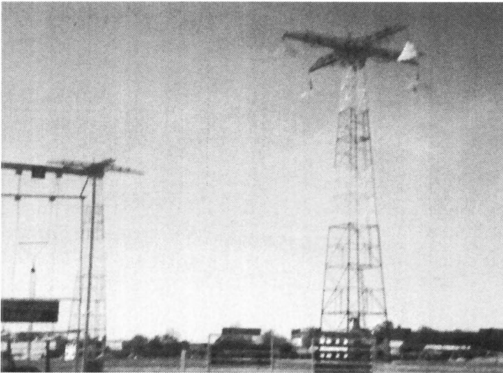
250' Jump Tower at Ft. Benning, GA
